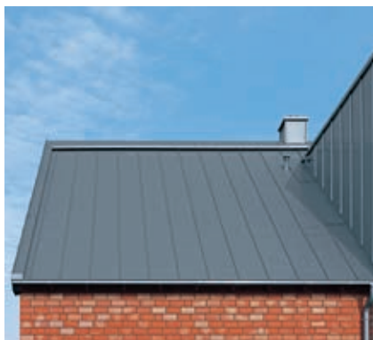
Standing seam covering with narrow gable coping and ventilated ridge
